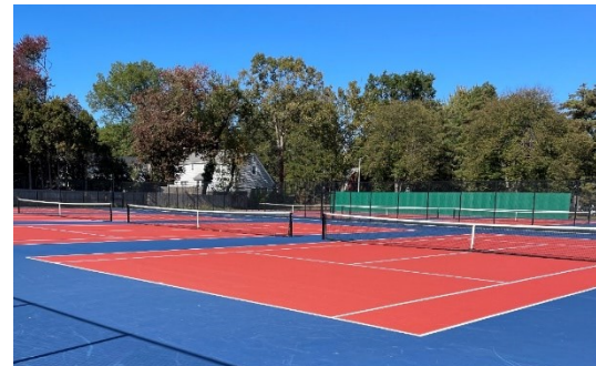
High School Tennis Court Replacement
