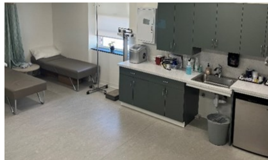
Middle School Nurses Office Renovation
