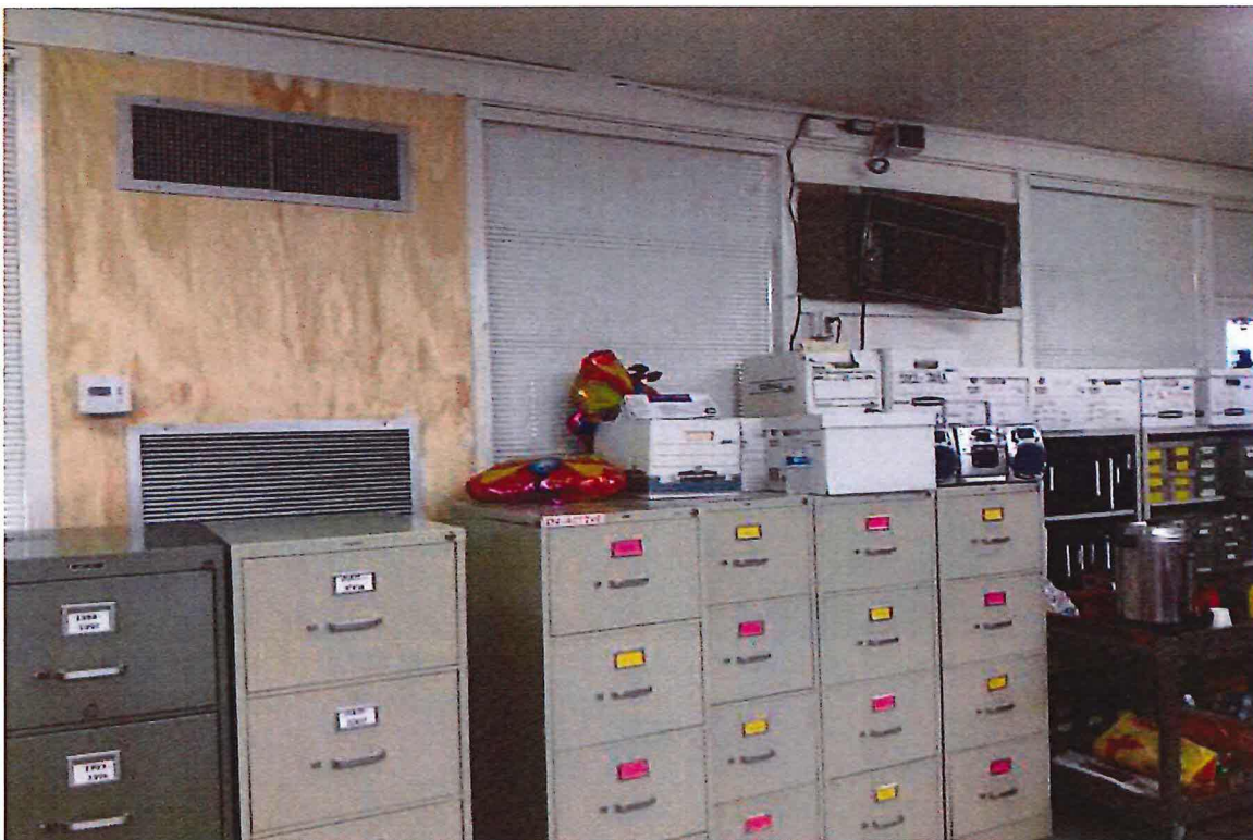
Vista HS – Interior Vent System (Old Window System to the Right)
