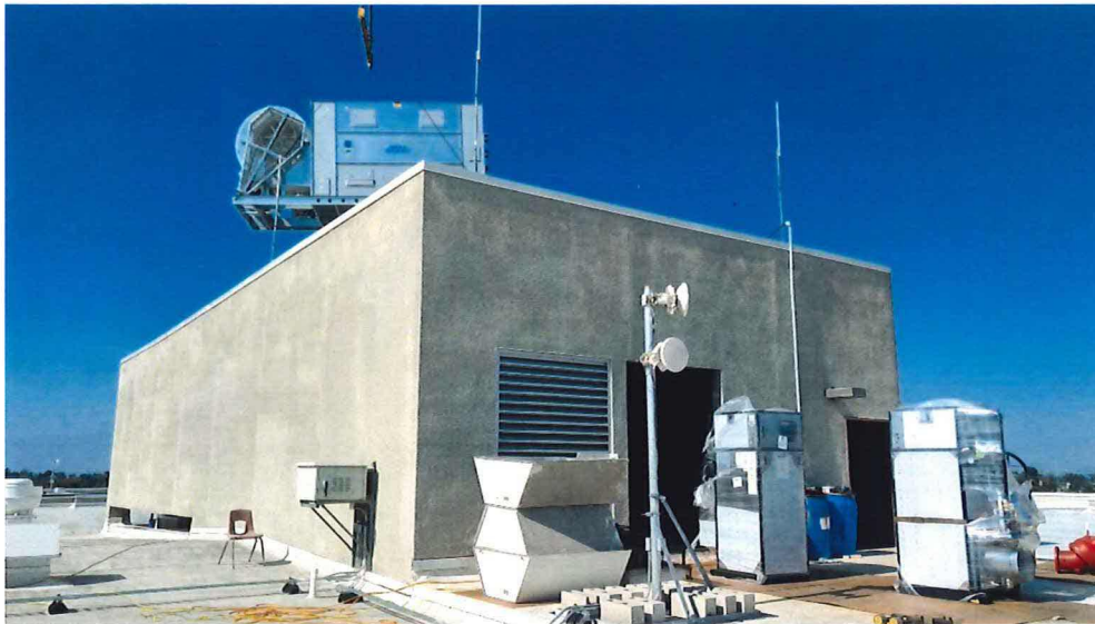
New tankless boilers and cooling towers craned to Mechanical Penthouse of 6000 wing
