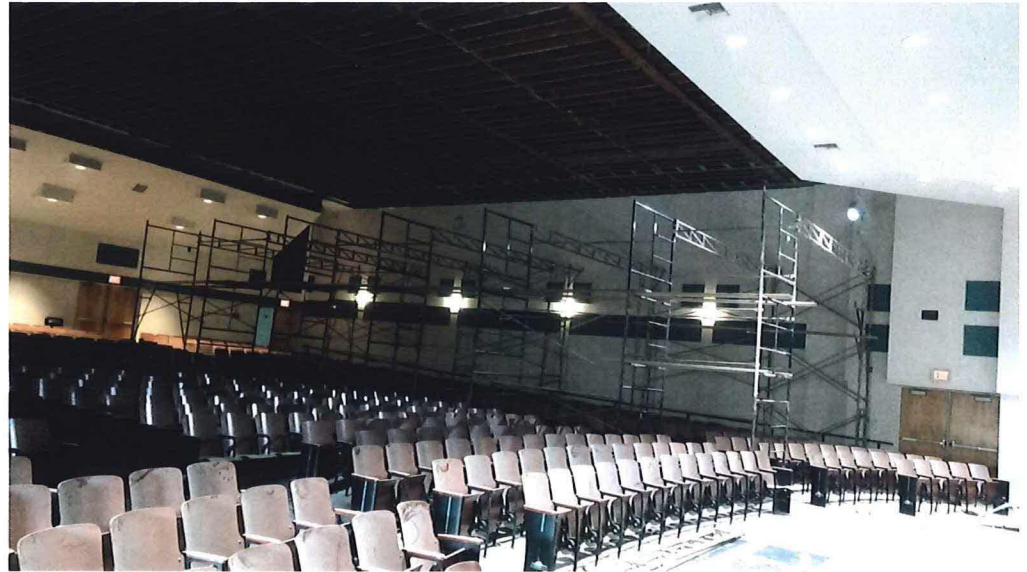
Ceiling removed Over Auditorium Seating
