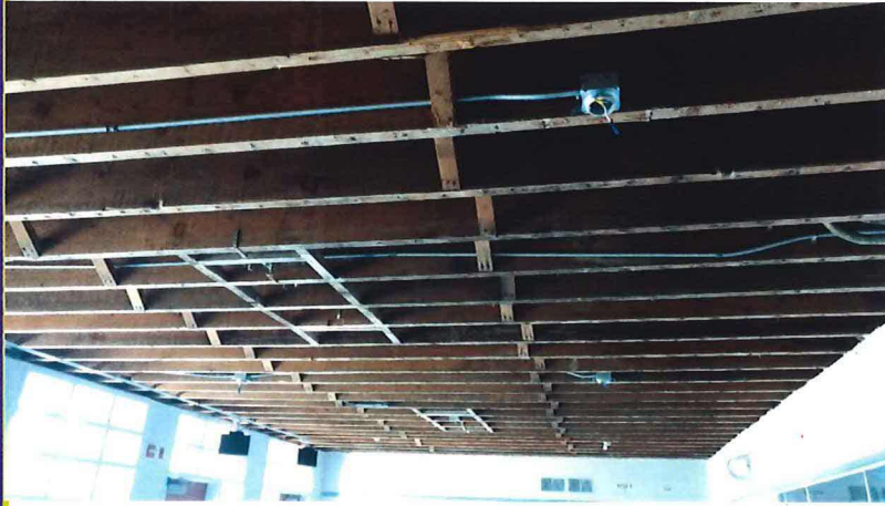
Ceiling Removed at Lobby
