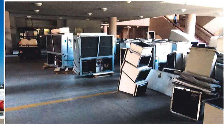
Old HVAC equipment removed from classrooms and labs in Classroom Building
