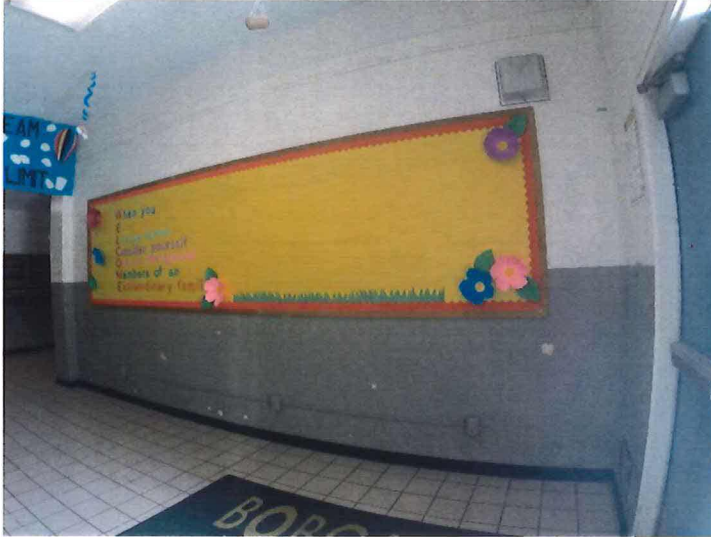
EXISTING ENTRANCE CORRIDOR
