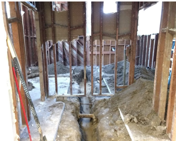
Reconstruction of Restrooms (During Construction)
