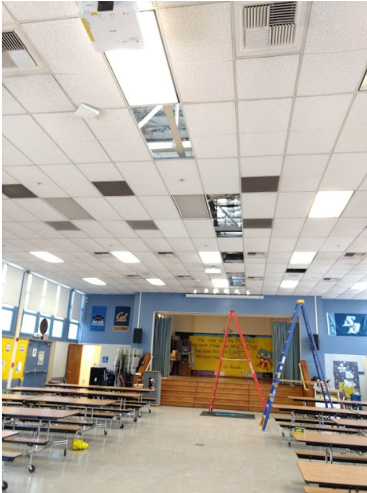
Conduit Installation above Rosa Parks Cafeteria Ceiling
