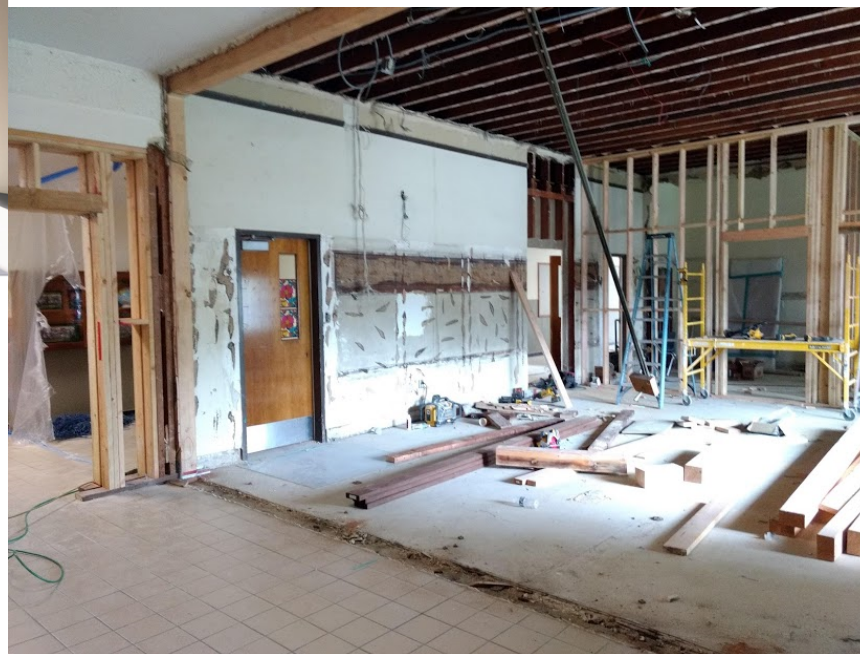
Photo during construction
