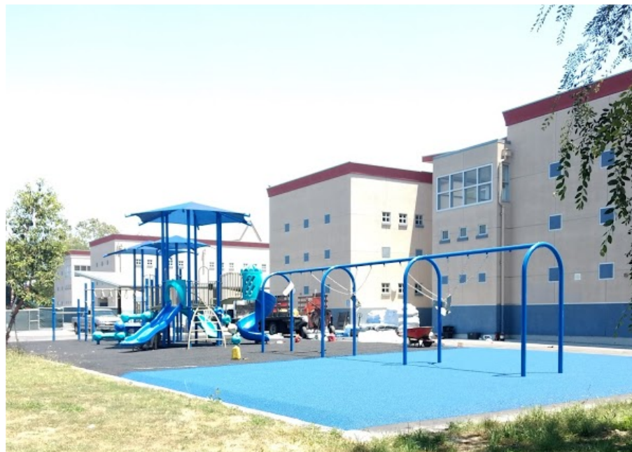
Primary Playground Equipment in final stages of construction
