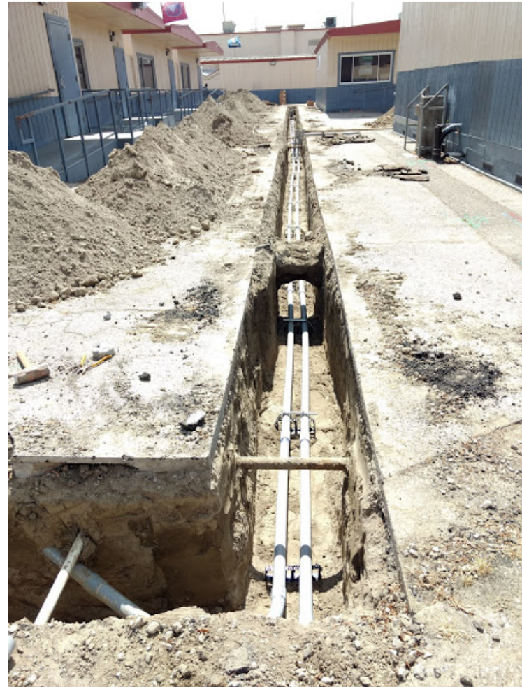
Underground Conduit Installation at Lynwood MS Portable Classrooms
