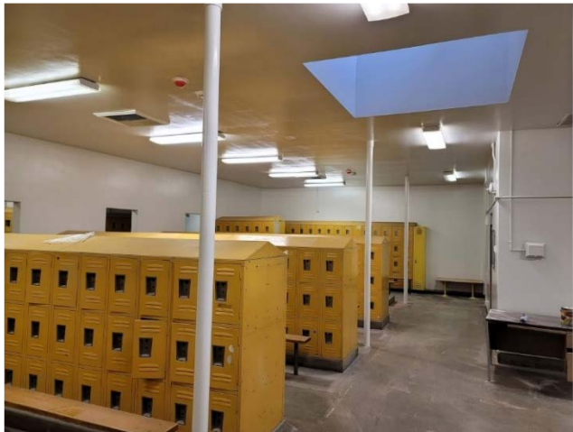
New Paint at Locker Rooms
