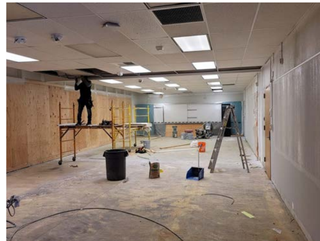
Construction of New Dance Room
