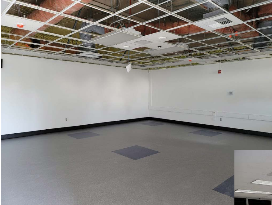
Refresh of Classroom Interiors In Progress
