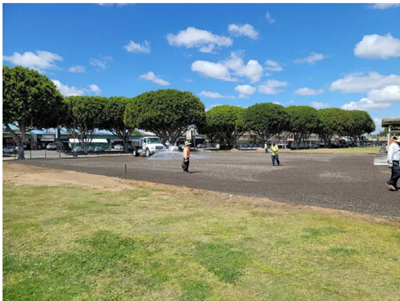
Placement of Asphalt Pad
