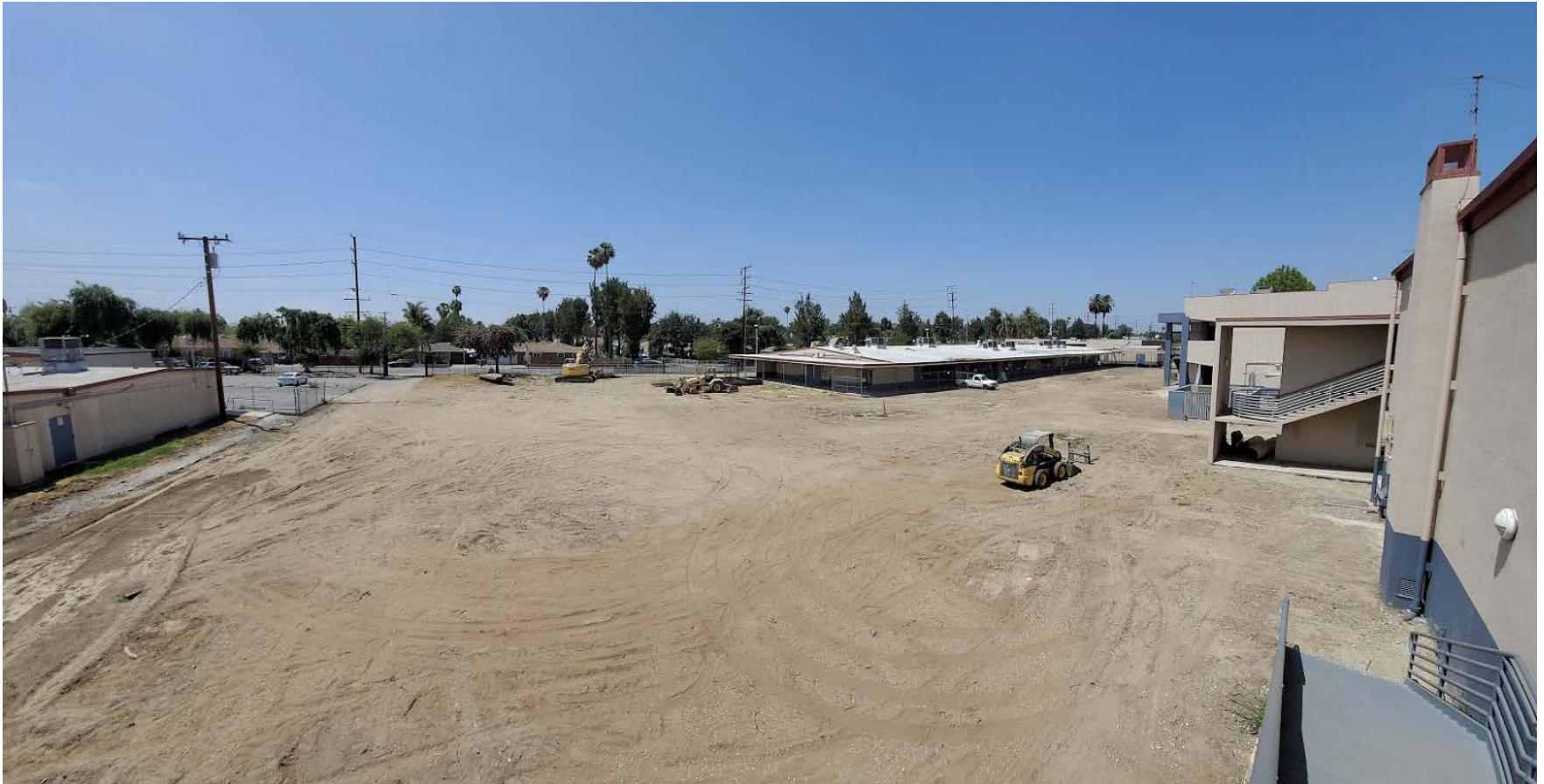
Site Clearing for New Quad and Staff Parking
