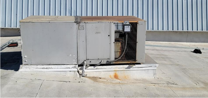
Will Rogers ES HVAC Replacement Project – Existing HVAC Unit scheduled for replacement
