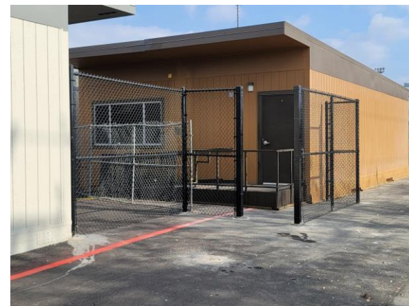
Fence Work at New Portable Classroom Building -- Lynwood HS Bullis
