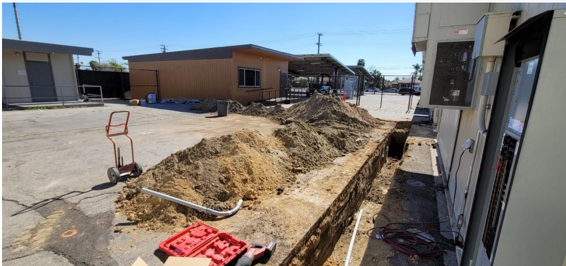
Data and Fire Alarm Infrastructure Work at New Portable Classroom Building -- Lynwood HS Bullis
