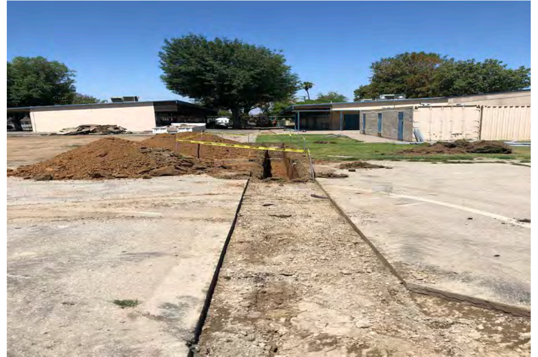
Trenching for future electrical service
