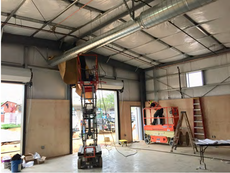
Ducting installation in progress, Interior Insulation complete. Electrical outlets and Disconnects installation in progress walls panels complete
