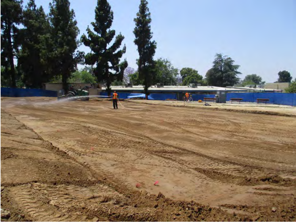
Grading sub-excavation and compaction is complete for the 5 relocated portables
