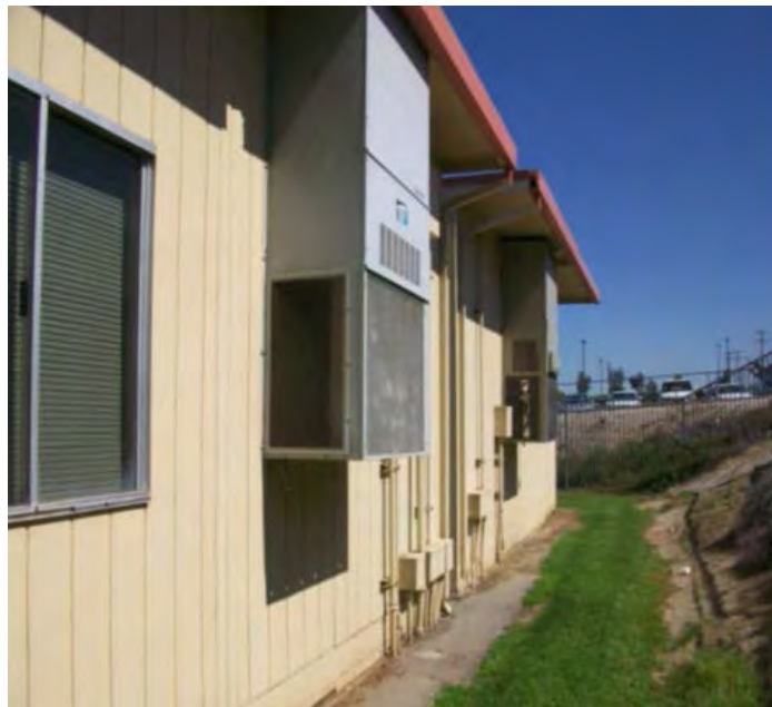
New High Efficiency and Quieter HVAC Unit
