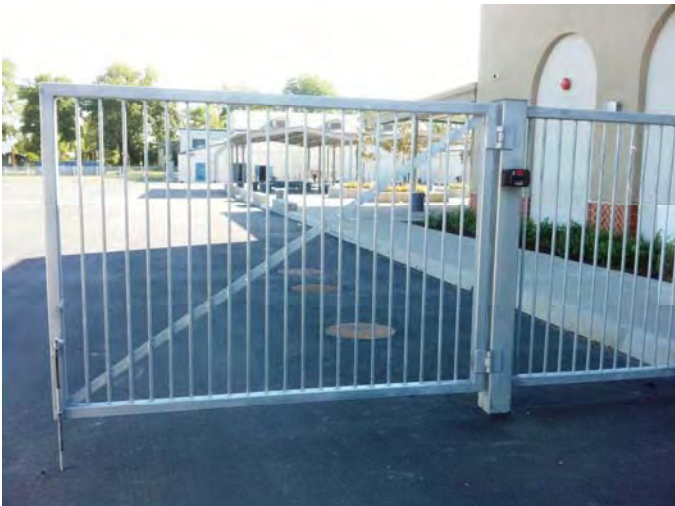
Fire lane drive gates can always be chained and padlocked, whether or not they have a "Knox Box" key vault.
