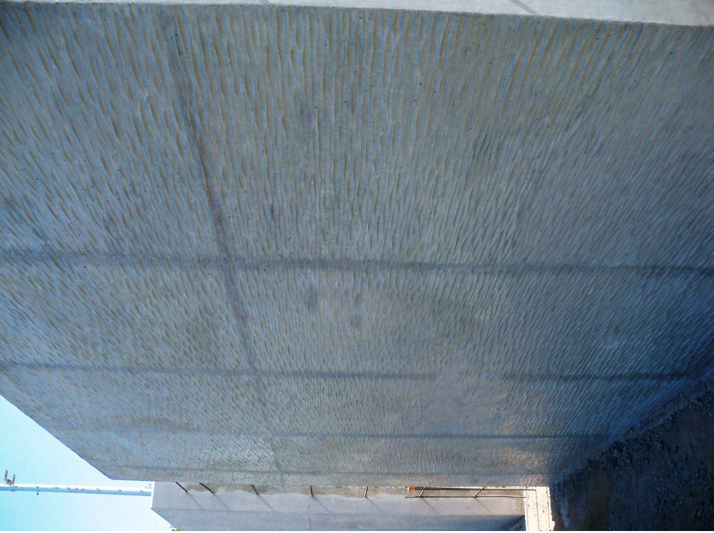
Wall form liner Detail
