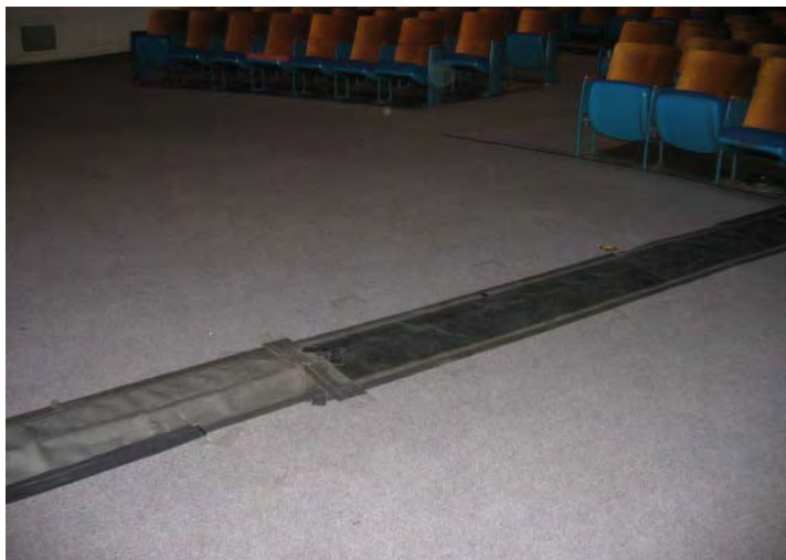
Surface mounted sound and light cabling
