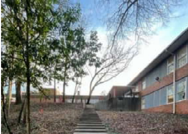
Building 5021 Stairs 2: Located adjacent to building 5021. Leads to the track and field.
