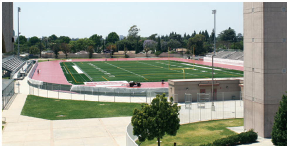
District Stadium renovation at Lynwood High.
