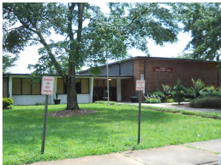
1). North Elevation - Jun 17, 2015
