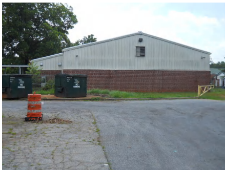
2). North Elevation - Jun 17, 2015
