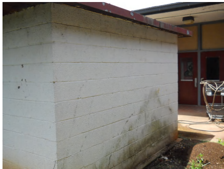
4). North Elevation - Jun 17, 2015
