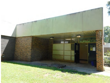
2). Southwest Elevation - Aug 12, 2015
