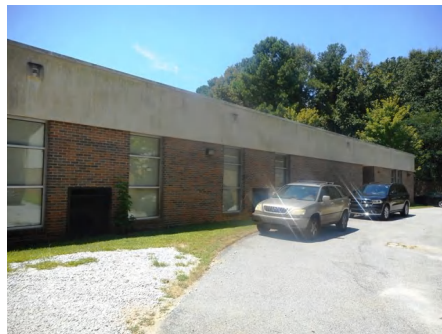
3). North Elevation - Aug 12, 2015
