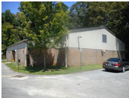
3). Southeast Elevation - Aug 12, 2015
