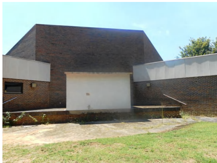
4). North Elevation - Aug 12, 2015
