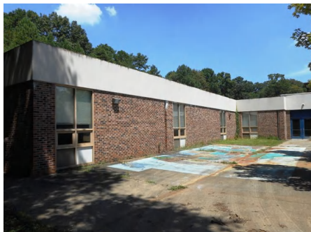
1). Southeast Elevation - Aug 12, 2015
