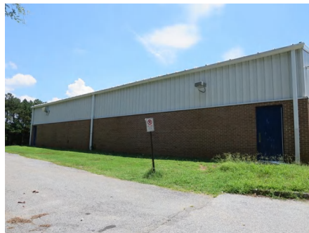
3). North Elevation - Jul 31, 2015
