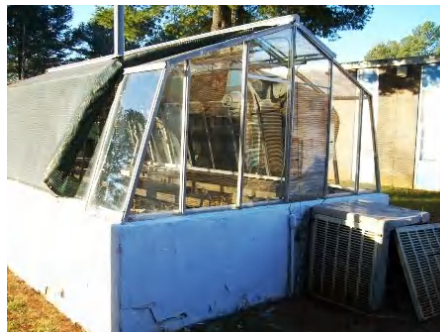
3). North Elevation - Dec 09, 2010
