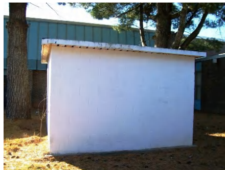
3). East Elevation - Jul 31, 2015
