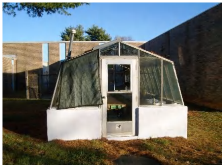
1). South Elevation - Dec 09, 2010
