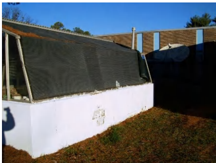
2). East Elevation - Dec 09, 2010
