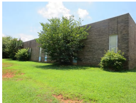
3). East Elevation - Jul 31, 2015
