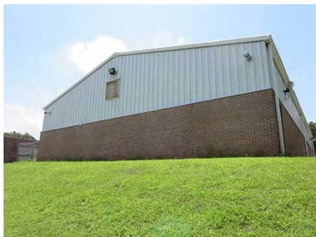
4). East Elevation - Jul 31, 2015
