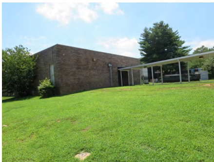
2). North Elevation - Jul 31, 2015
