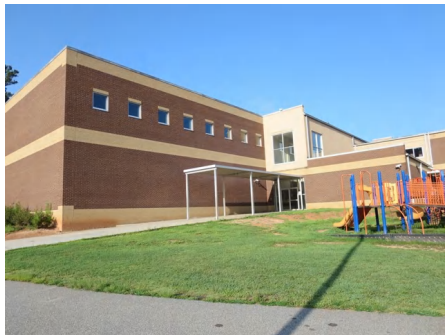
4). North Elevation - Jul 29, 2015
