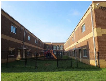
5). North Elevation - Jul 29, 2015
