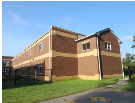
6). North Elevation - Jul 29, 2015
