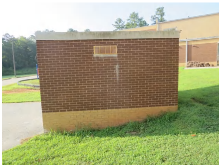
2). North Elevation - Jul 29, 2015
