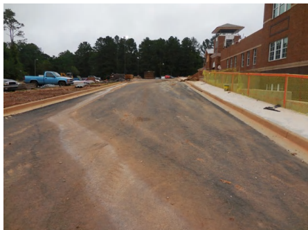
1). Site Under Construction - Jul 06, 2015
