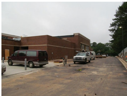
4). North Elevation - Jul 06, 2015
