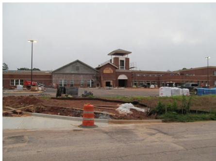
1). East Elevation - Jul 06, 2015
