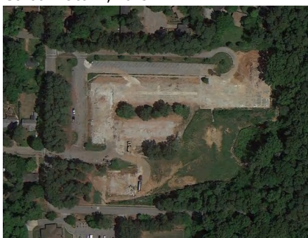
5). Aerial Image of Peachcrest Elementary School - Oct 22, 2015
