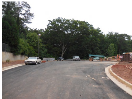
3). Site Under Construction - Jul 06, 2015
