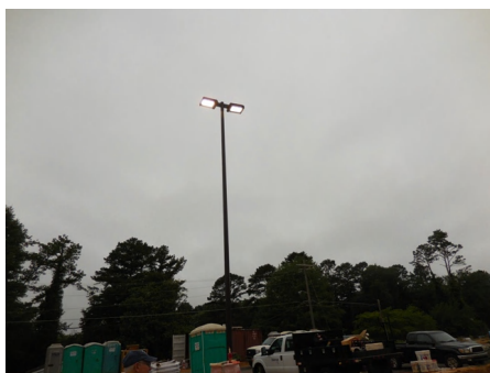
4). Site Under Construction - Jul 06, 2015
