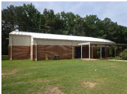
1). North Elevation - Jul 08, 2015
