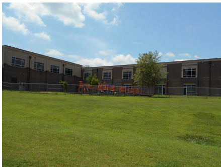
2). North Elevation - Jul 29, 2015
