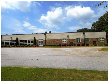
4). East Elevation - Jul 24, 2015
