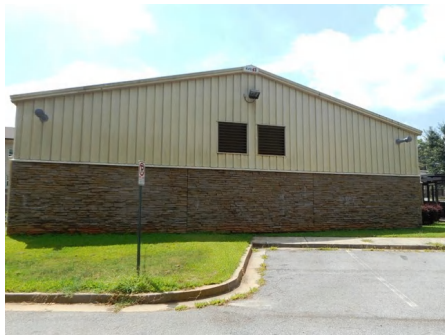
4). North Elevation - Jul 24, 2015
