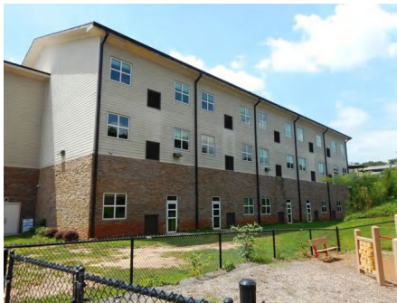
5). Northeast Elevation - Jul 24, 2015
