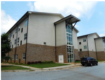
2). Southeast Elevation - Jul 24, 2015
