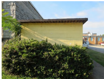
3). North Elevation - Aug 12, 2015
