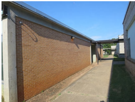
4). North Elevation - Aug 12, 2015
