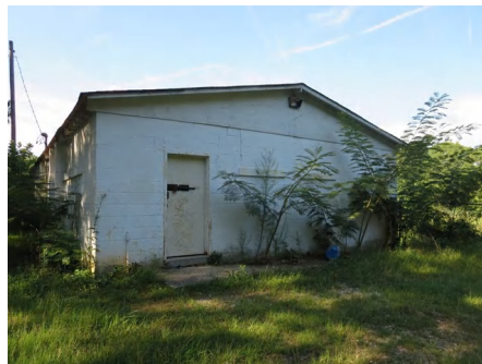
3). North Elevation - Aug 12, 2015
