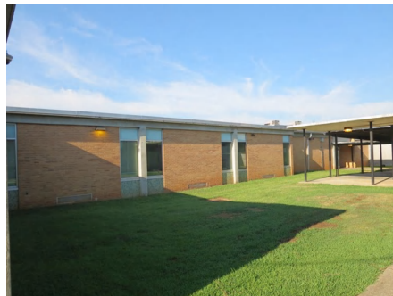
3). North Elevation - Aug 12, 2015
