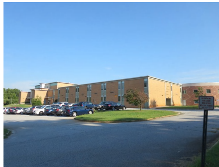
6). Southeast Elevation - Aug 12, 2015
