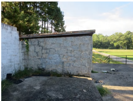
2). North Elevation - Aug 12, 2015
