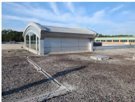
4). North Roof Elevation - Aug 12, 2015
