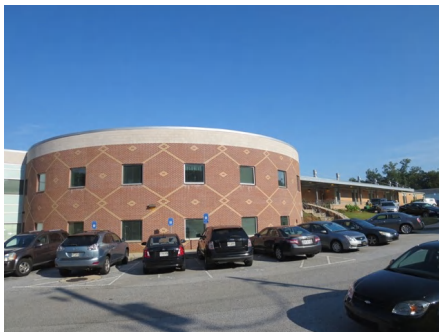
2). Southeast Elevation - Aug 12, 2015
