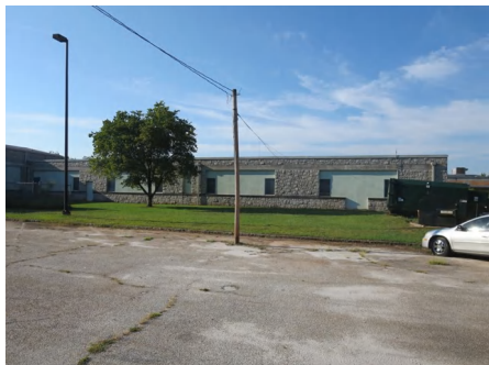
1). North Elevation - Aug 11, 2015
