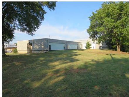
3). Northeast Elevations - Aug 11, 2015
