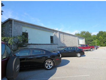
4). North Elevation - Aug 11, 2015
