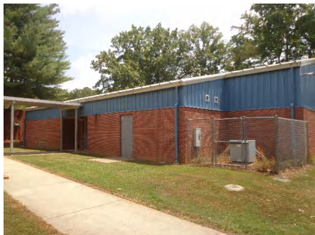
1). North Elevation - Aug 03, 2015
