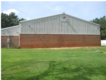
2). North Elevation - Jul 14, 2015
