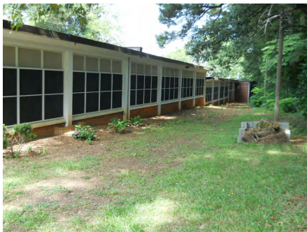
2). North Elevation - Jul 14, 2015
