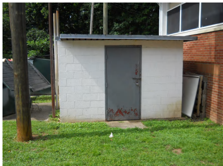
1). North Elevation - Jul 14, 2015
