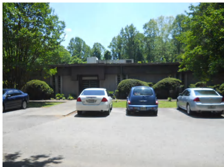
1). North Elevation - May 12, 2015
