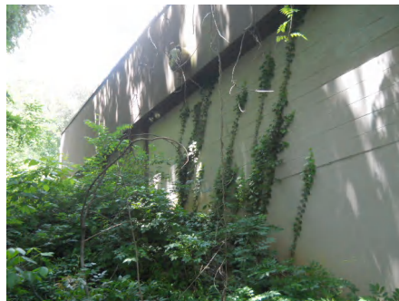
3). South Elevation - May 12, 2015
