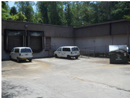
4). East Elevation - May 12, 2015
