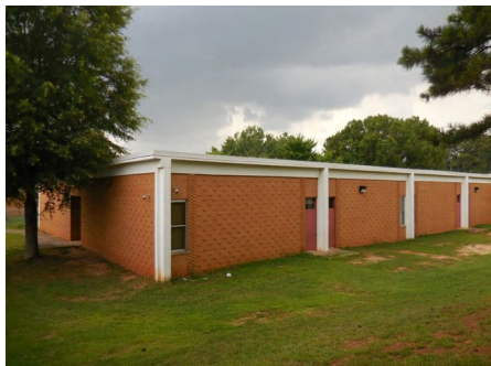
1). North Elevation - Jul 01, 2015
