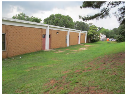
3). North Elevation - Jul 01, 2015
