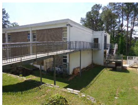
6). North Elevation - May 04, 2015
