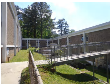
5). North Elevation - Courtyard - Apr 30, 2015
