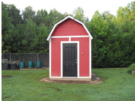
1). North Elevation - Jul 08, 2015
