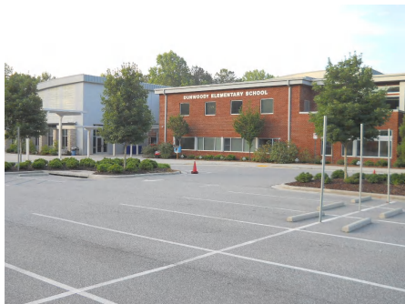
1). North Elevation - Jul 08, 2015
