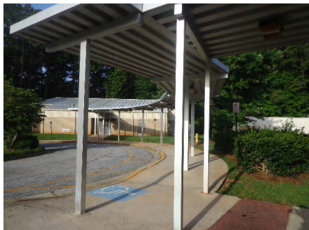
1). Covered Walkways - Jun 30, 2015
