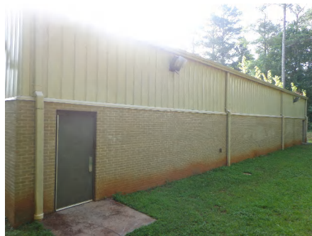
3). Southwest Elevation - Jul 01, 2015
