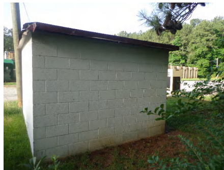
3). North Elevation - Jun 29, 2015
