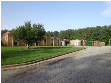
4). North Elevation - Jun 29, 2015
