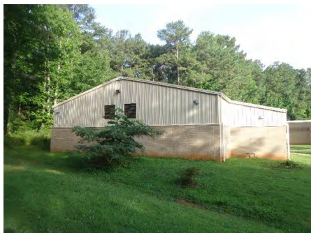
4). Southeast Elevation - Jul 01, 2015
