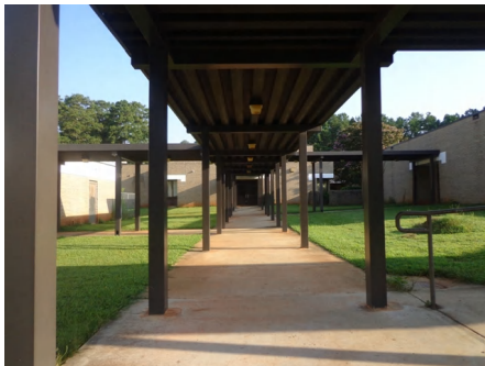
2). Covered Walkway - Jul 20, 2015
