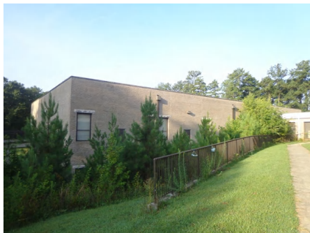
1). North Elevation - Jul 20, 2015
