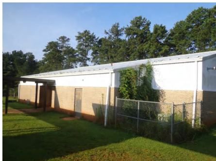
1). Northeast Elevation - Jul 20, 2015
