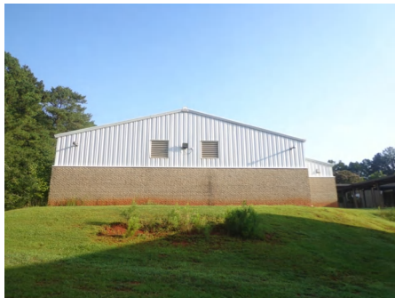
4). Southeast Elevation - Jul 20, 2015
