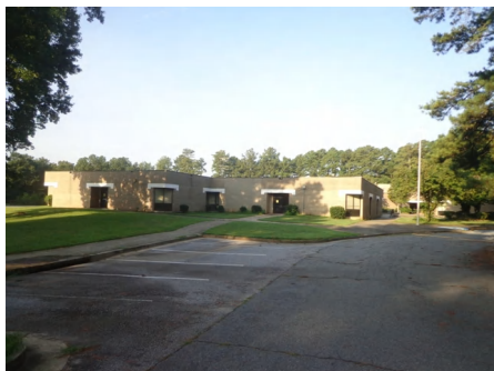
4). Northeast Elevation - Jul 20, 2015
