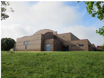
2). North Elevation - Jun 05, 2015
