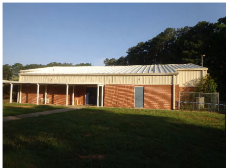
1). East Elevation - Jul 02, 2015
