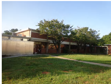
3). Northeast Elevation - Jul 04, 2015
