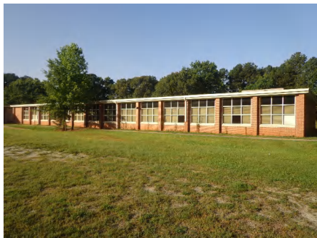
1). Northeast Elevation - Jul 02, 2015
