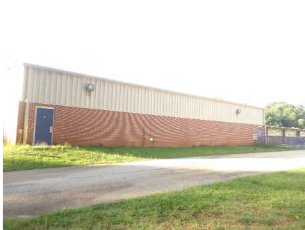
2). North Elevation - Jul 02, 2015
