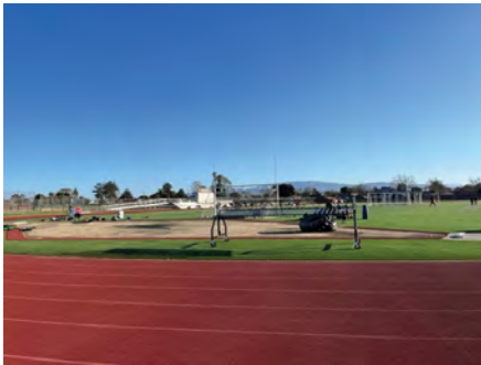
② Looking south from northern portion of stadium site.
