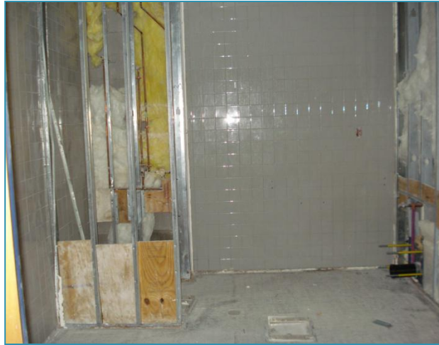
NEW BATHROOM TILE
