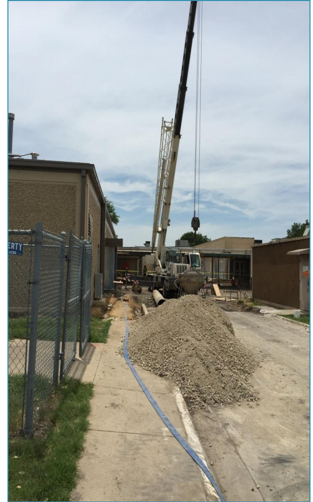
GRADE PREP FOR THE ADDITION
