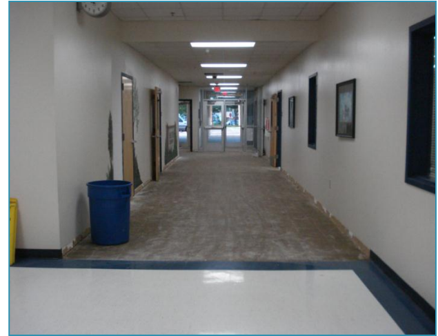
NEW MAIN ENTRY TILE
