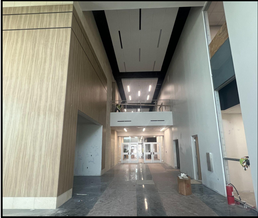
Main Entry Corridor and Reception
