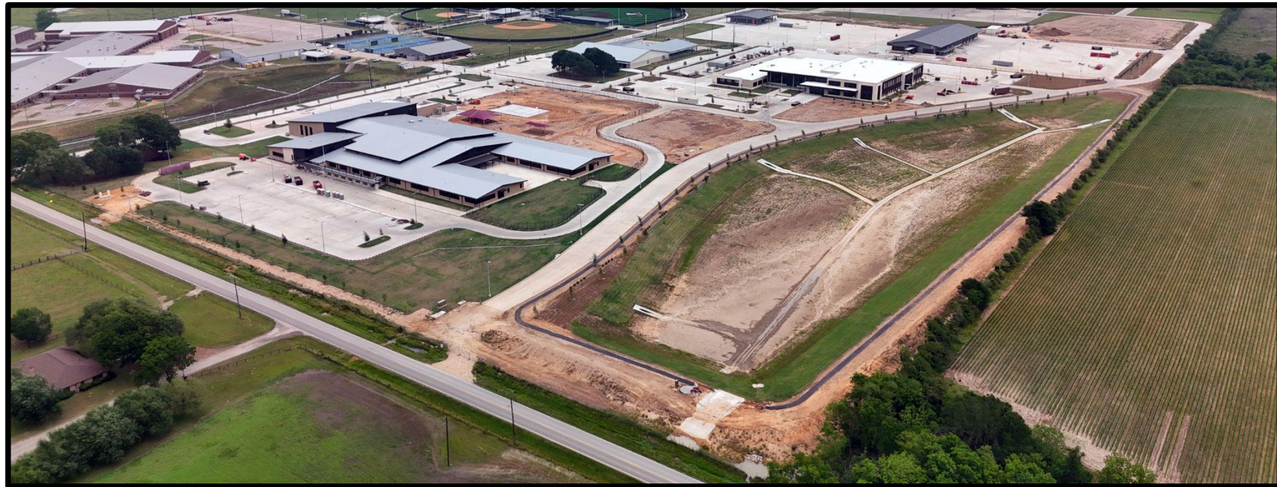
Aerial View - Southwest Corner (February 2025)
