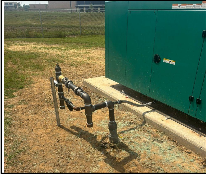
Schultz Generator Install
