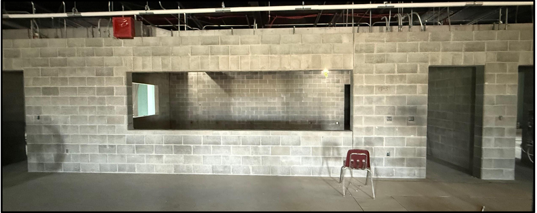
WJH Field House Reno
