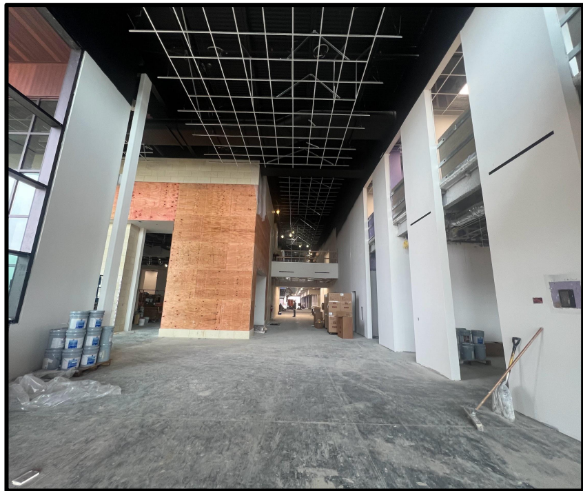
Main Entry Corridor and Reception
