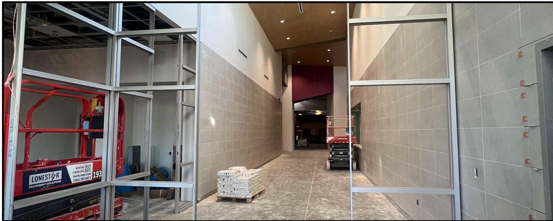
Front Entry Corridor
