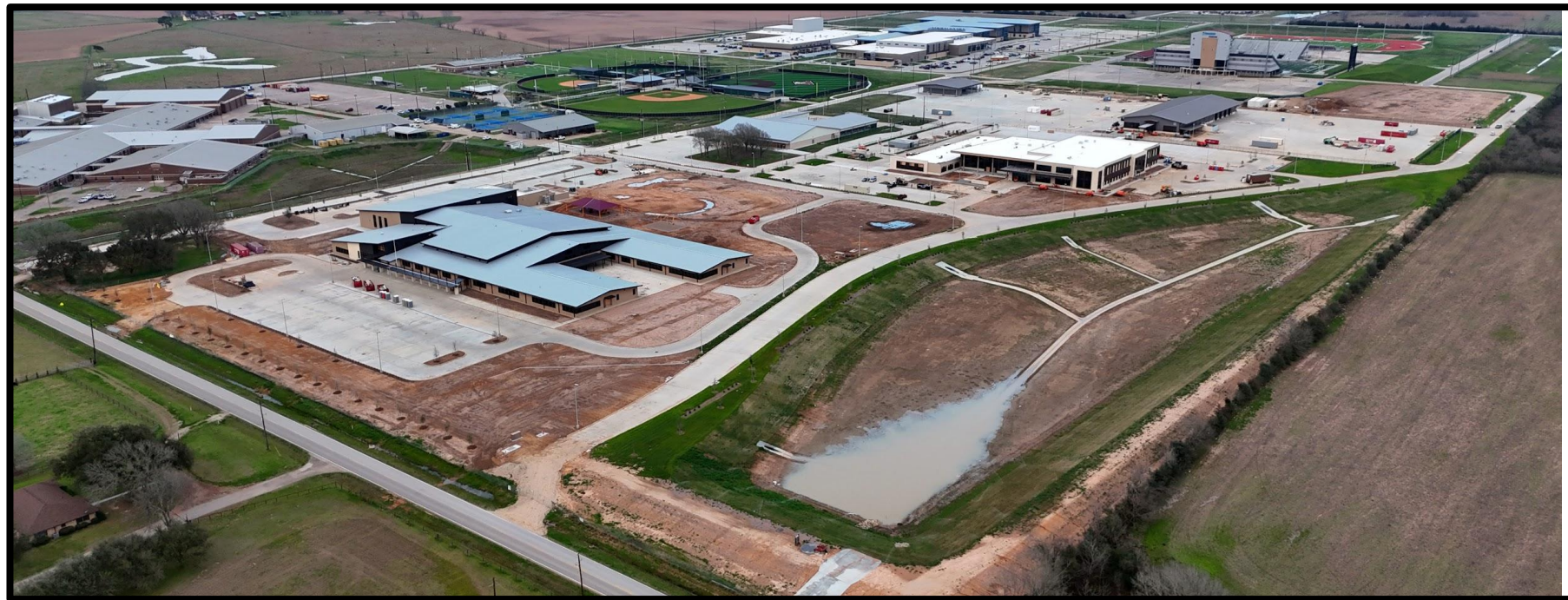
Aerial View - Southwest Corner (February 2025)
