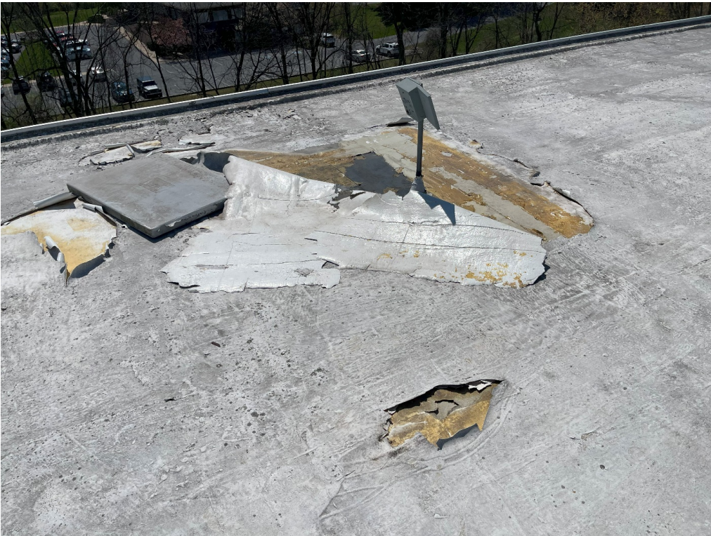
Roofing Delamination
