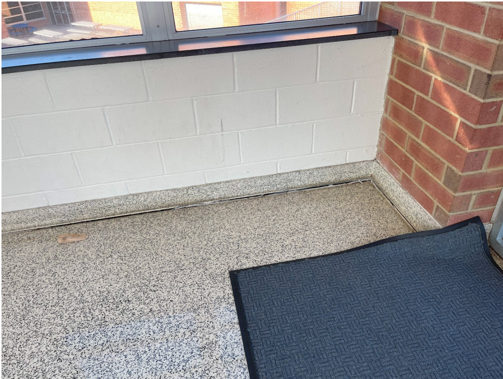
Settling & Cracking
