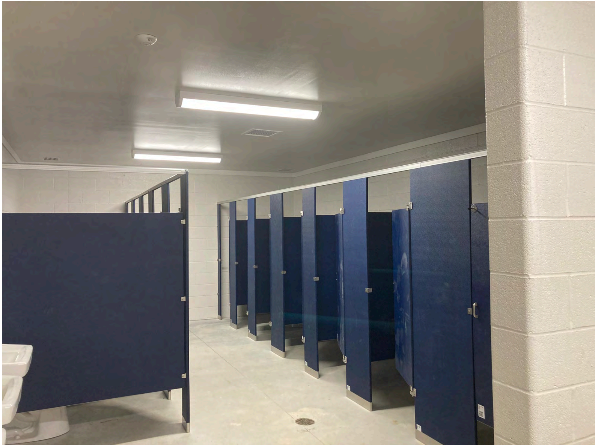
PERRYVILLE HIGH SCHOOL – FIELDHOUSE
