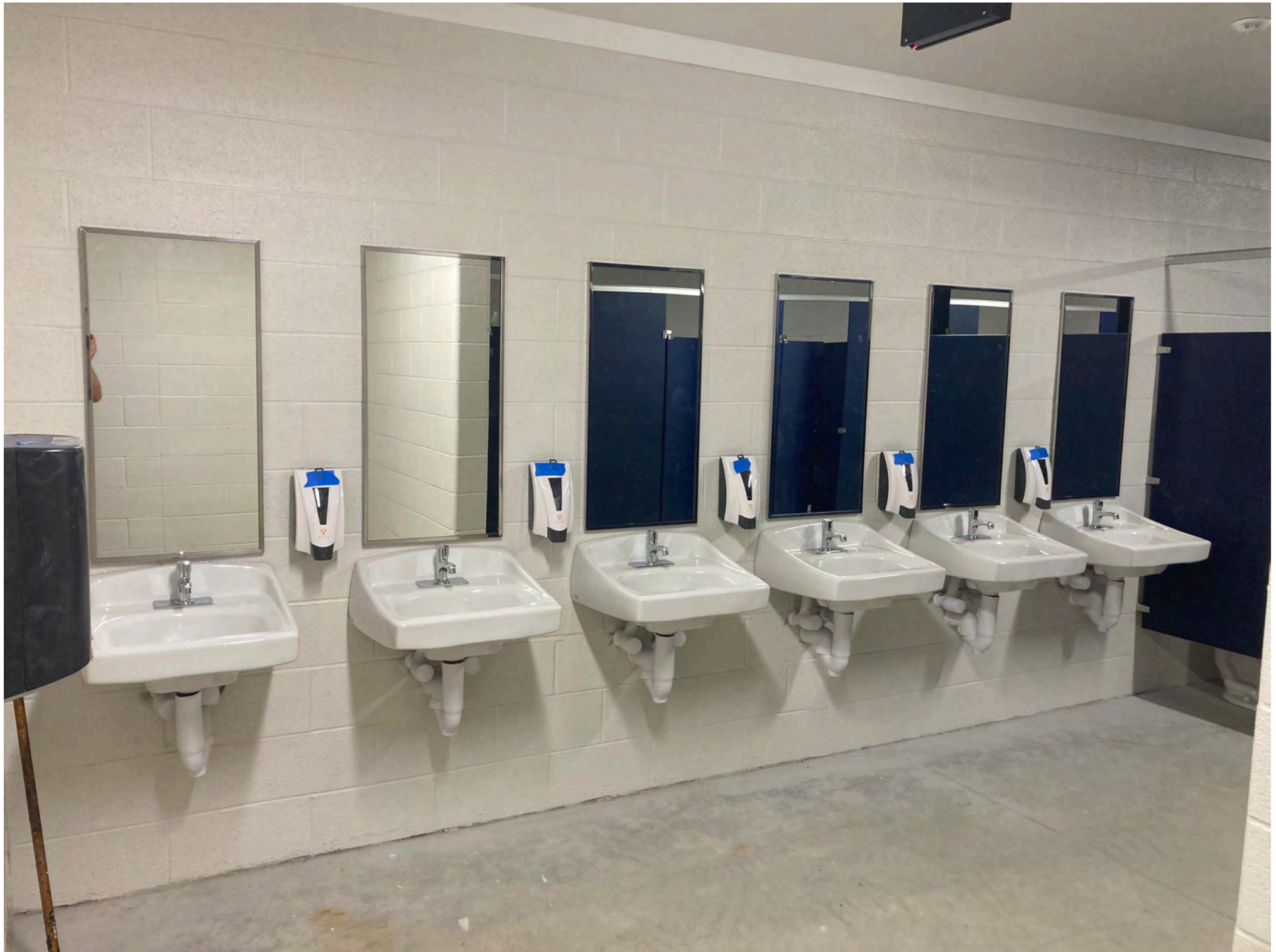
PERRYVILLE HIGH SCHOOL – FIELDHOUSE
