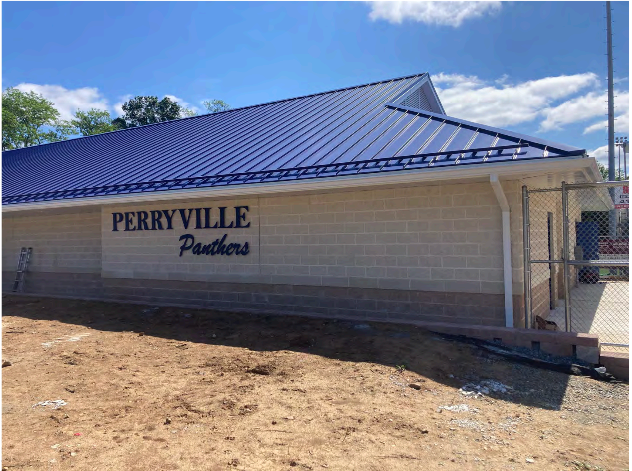
PERRYVILLE HIGH SCHOOL – FIELDHOUSE
