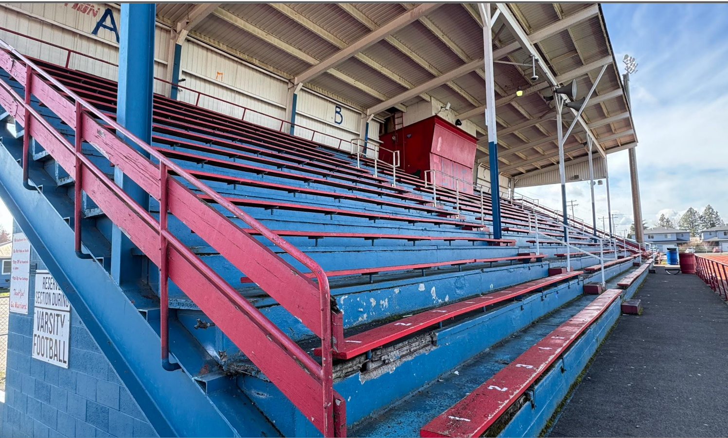
Heath Stadium Grandstands view
