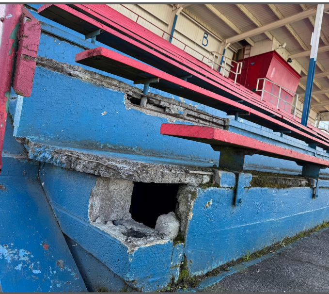
Exposed rebar steel reinforcing rod for the concrete
