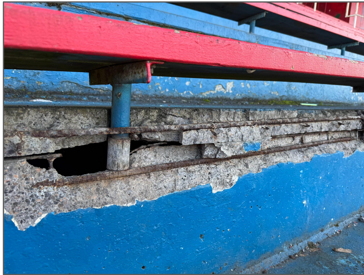
Exposed rebar steel reinforcing rod for the concrete
