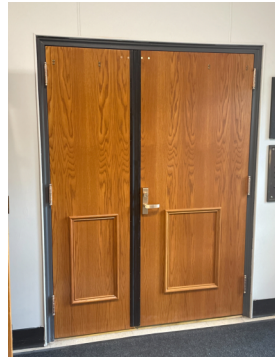
SDS - New auditorium doors and hardware installed
