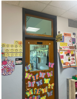
SDS - Security film installed on interior door lites
