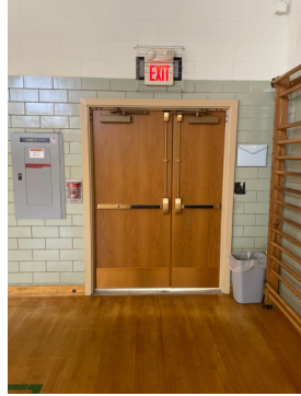
WBS - New gym and auditorium doors and hardware installed
