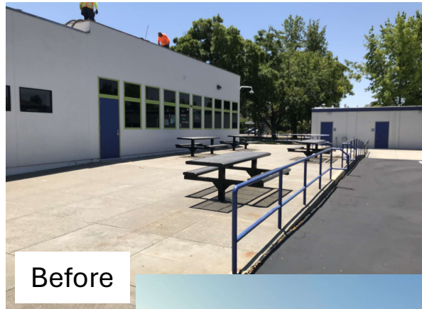
Arroyo Seco Shade Structure
