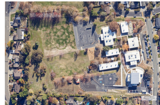
Blanche Sprentz Elementary School New Multipurpose Building
