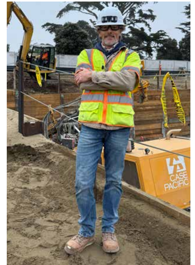
Brent Wheeler '82 on the New Learning Commons construction site
