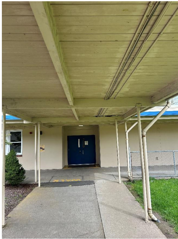
Metal downspout sampling locations
