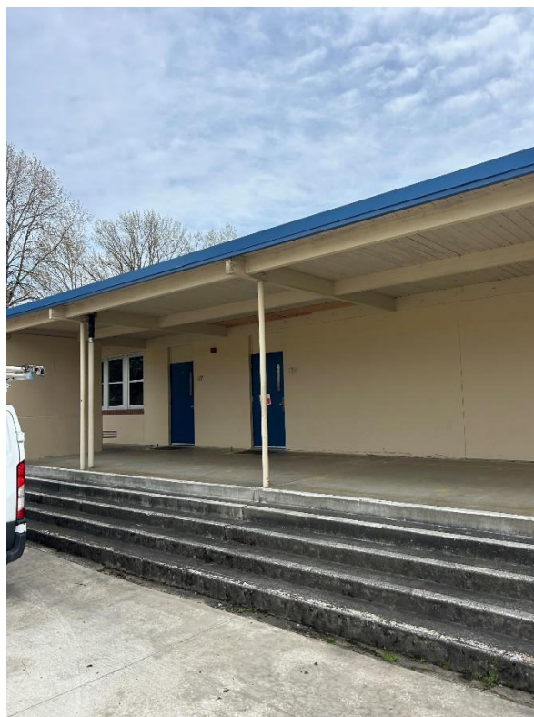
Ceiling area under roof eave
