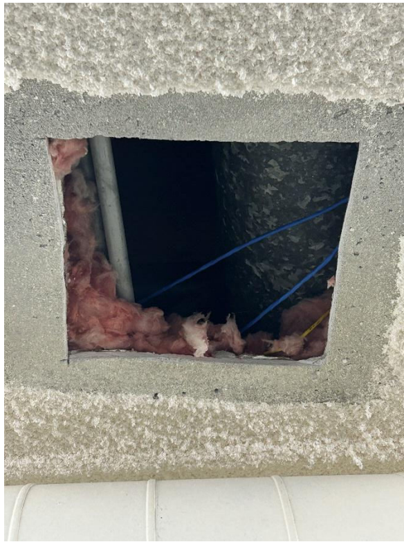
Ceiling area opening after HVAC upgrade
