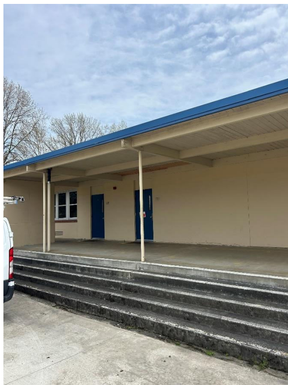
Ceiling area under roof eave
