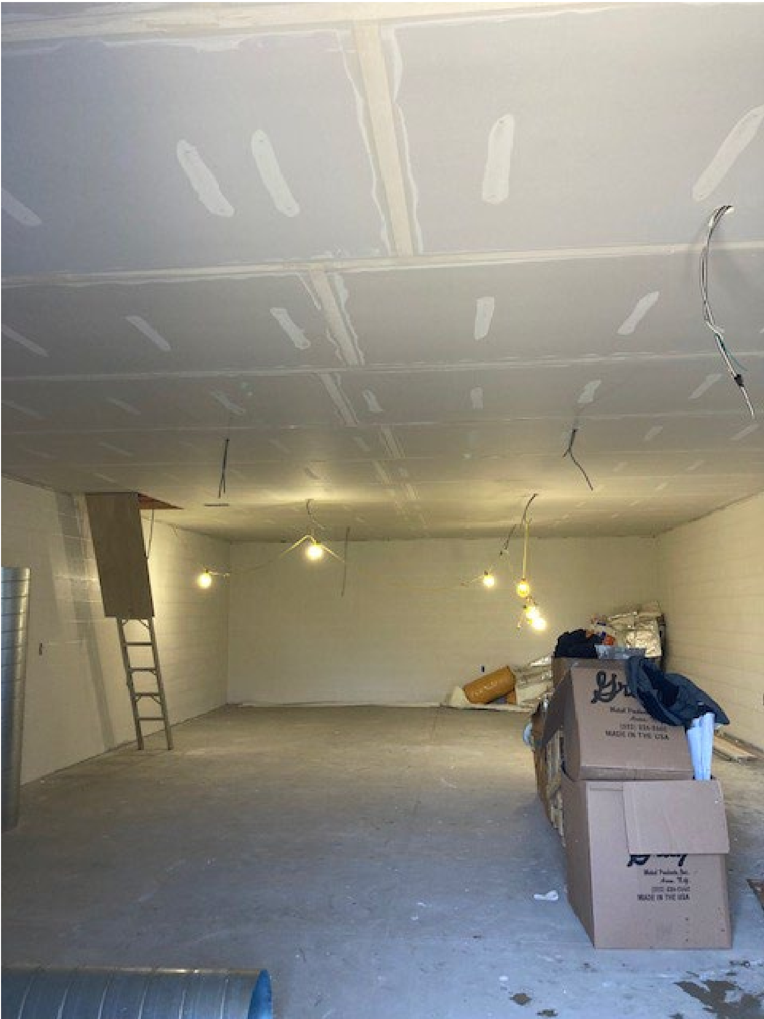
PERRYVILLE HIGH SCHOOL - FIELDHOUSE
