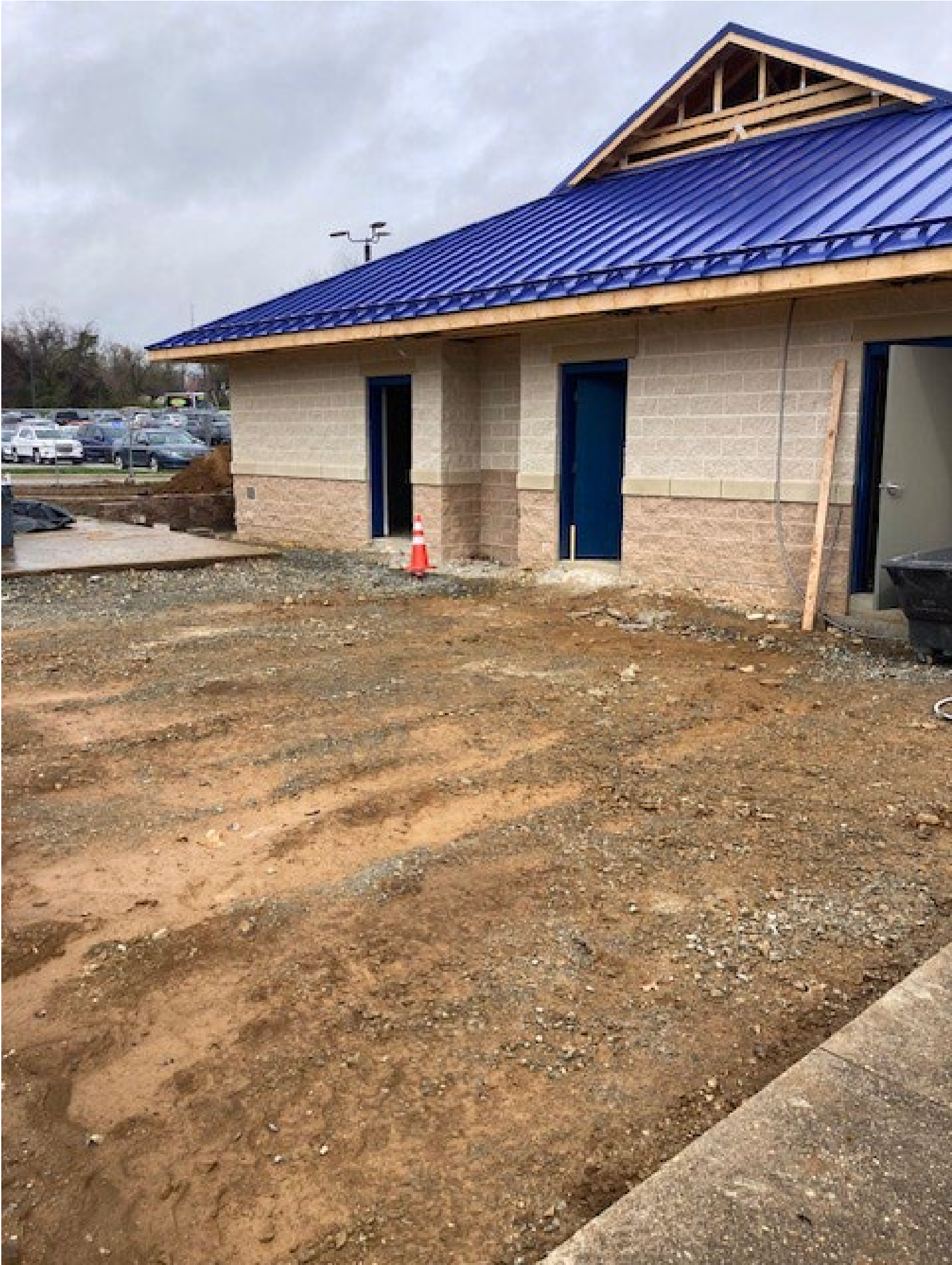
PERRYVILLE HIGH SCHOOL – FIELDHOUSE
