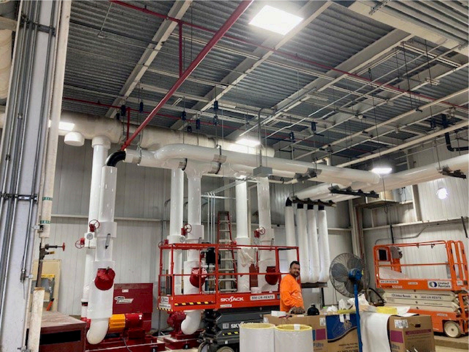
CECIL COUNTY SCHOOL OF TECHNOLOGY – CHILLER REPLACEMENT
