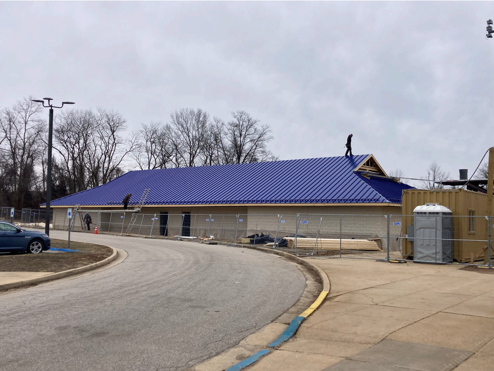
PERRYVILLE HIGH SCHOOL – FIELDHOUSE
