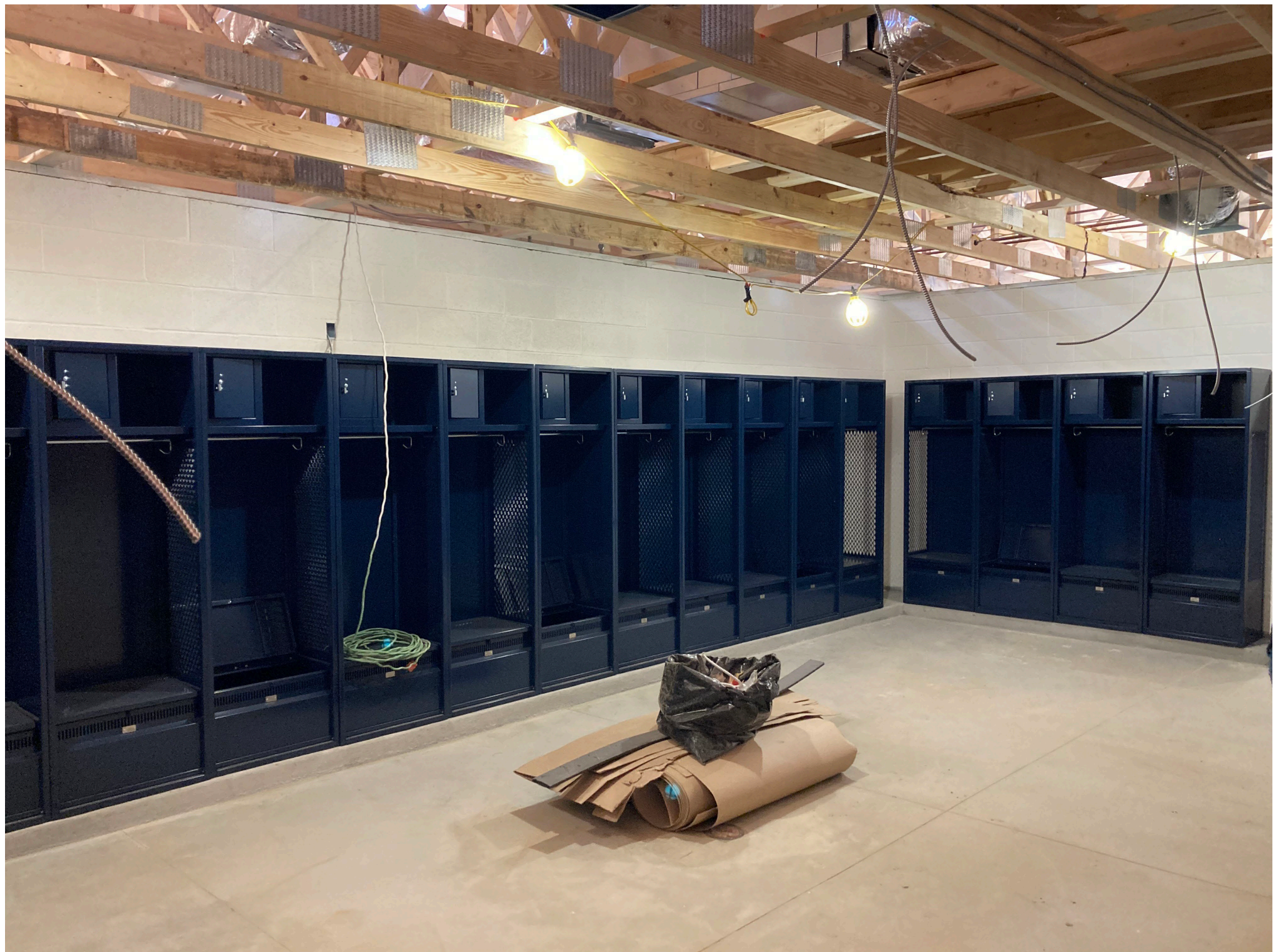
PERRYVILLE HIGH SCHOOL – FIELDHOUSE
