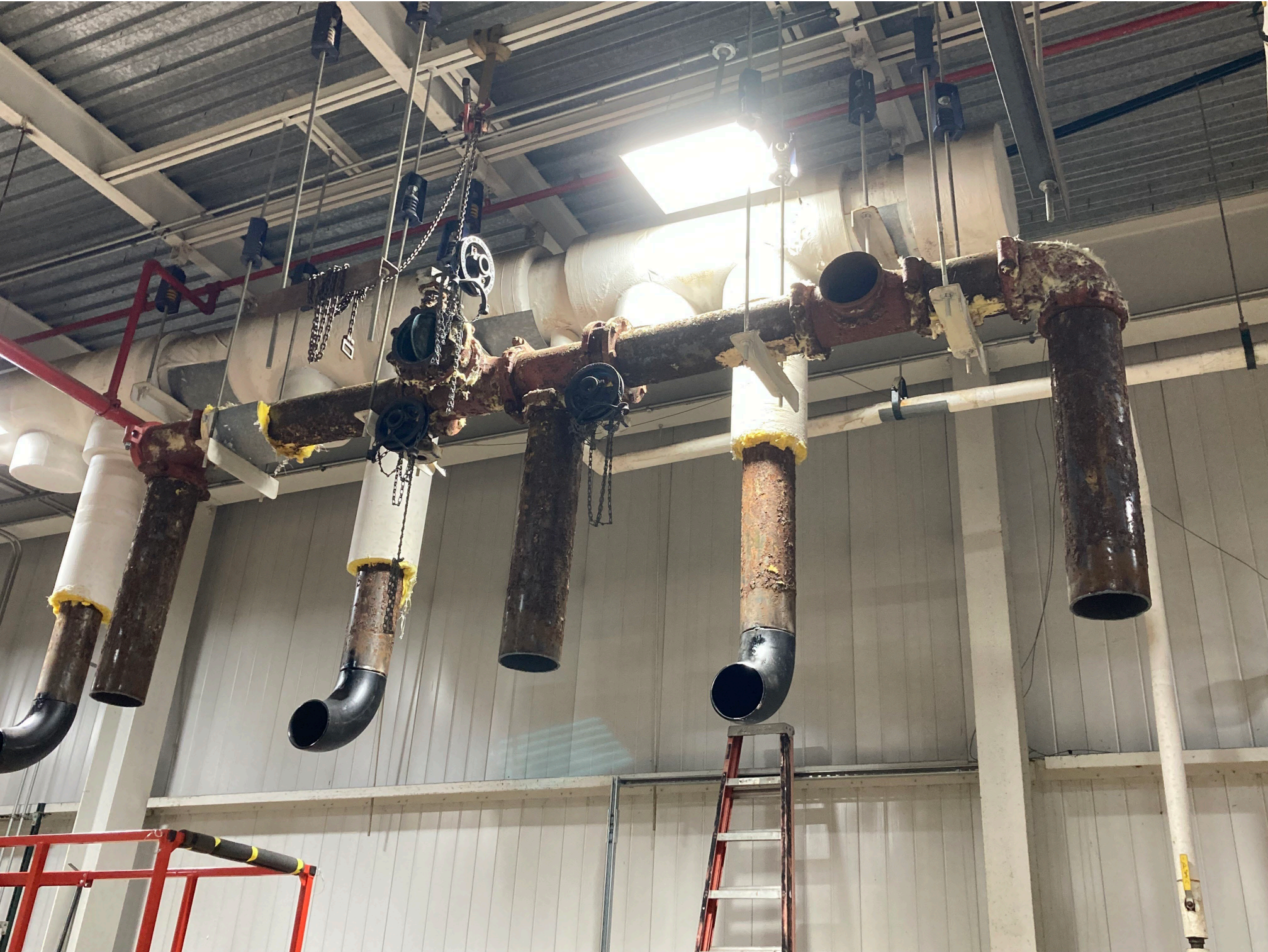
CECIL COUNTY SCHOOL OF TECHNOLOGY – CHILLER REPLACEMENT
