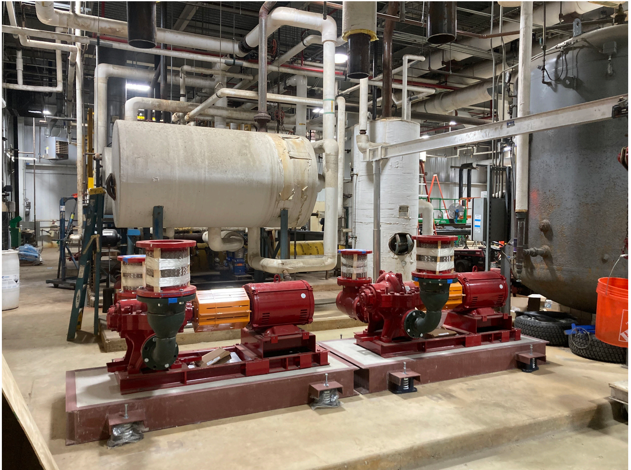
CECIL COUNTY SCHOOL OF TECHNOLOGY – CHILLER REPLACEMENT
