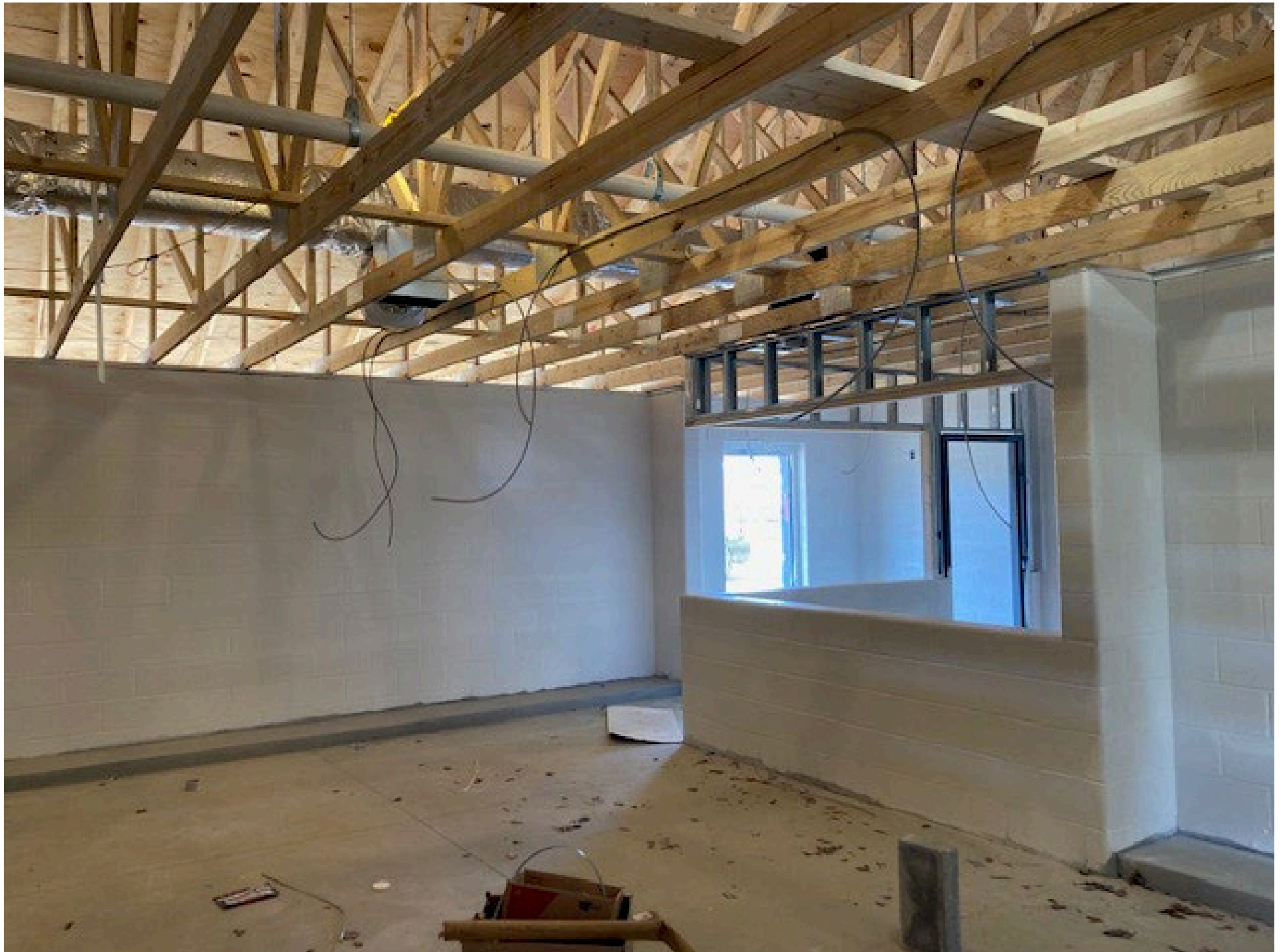
PERRYVILLE HIGH SCHOOL – FIELDHOUSE
