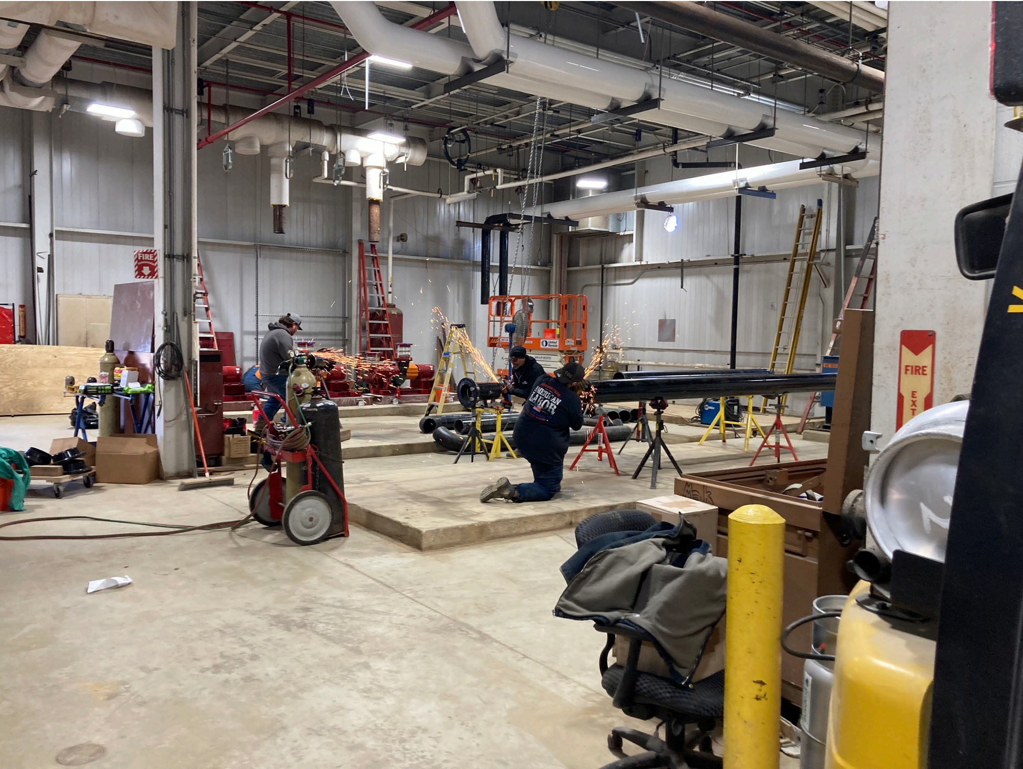
CECIL COUNTY SCHOOL OF TECHNOLOGY – CHILLER REPLACEMENT
