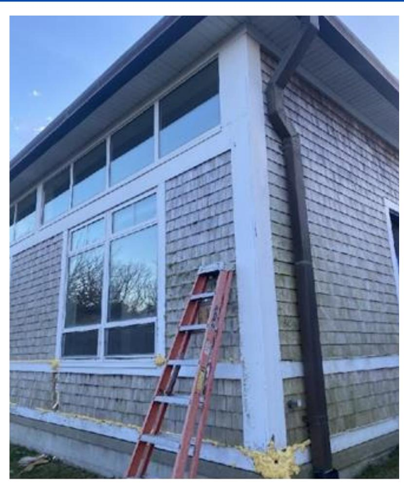
Spray foam insulation used to keep rainwater out
