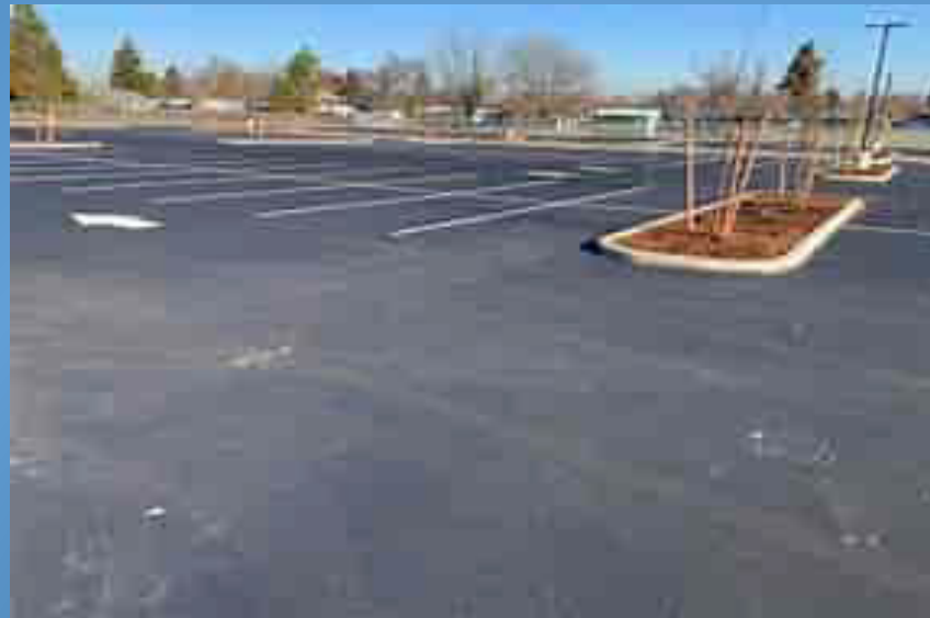
Parking Lot Improvements
