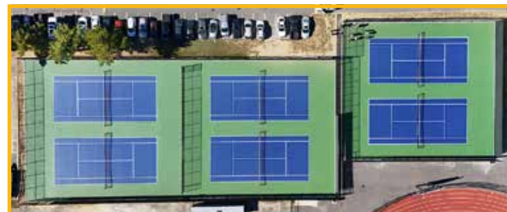
The high school tennis courts have been completely replaced, including surrounding fencing, while the four courts at Reed School received renovations last summer.
