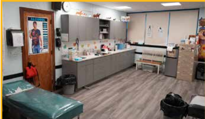
Nurse stations at Morrow and Cordello were renovated. Se renovaron las estaciones de enfermería en Morrow y Cordello.
